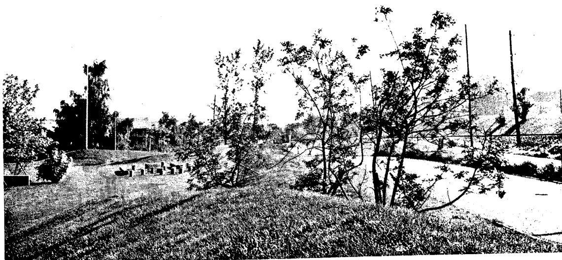
48 & 49 Surplus excavated material is moulded to pleasing landform providing privacy by visual screening and acoustic baffling from adjoining traffic and train noise. Zurich. p.47, para. 97.
