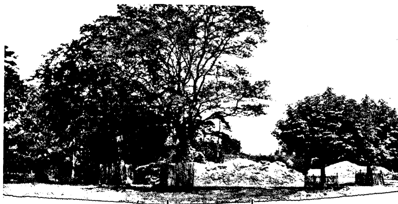
51 Top soil removed from building curtilage (pegs show position of building) and stacked in background. Chestnut paling to protect the trees should be noted. Illustration 53 shows the same site after development. Crawley, Sussex. p.48, para. 95 and 98.
