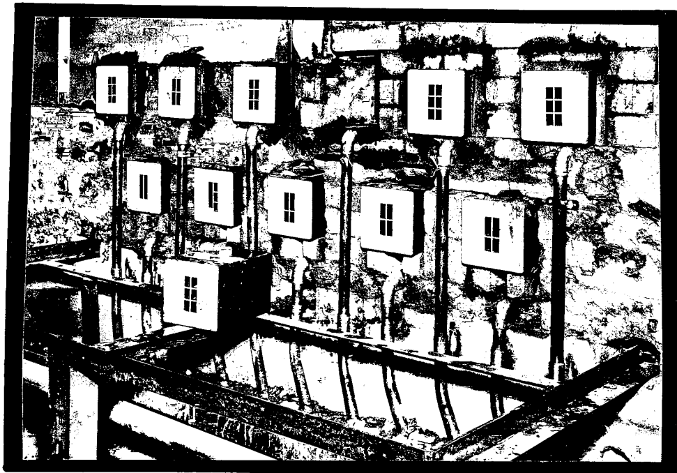
LEAD LINED STEEL BOXES WITH DRAWER HOLES & EVACUATION SYSTEM
